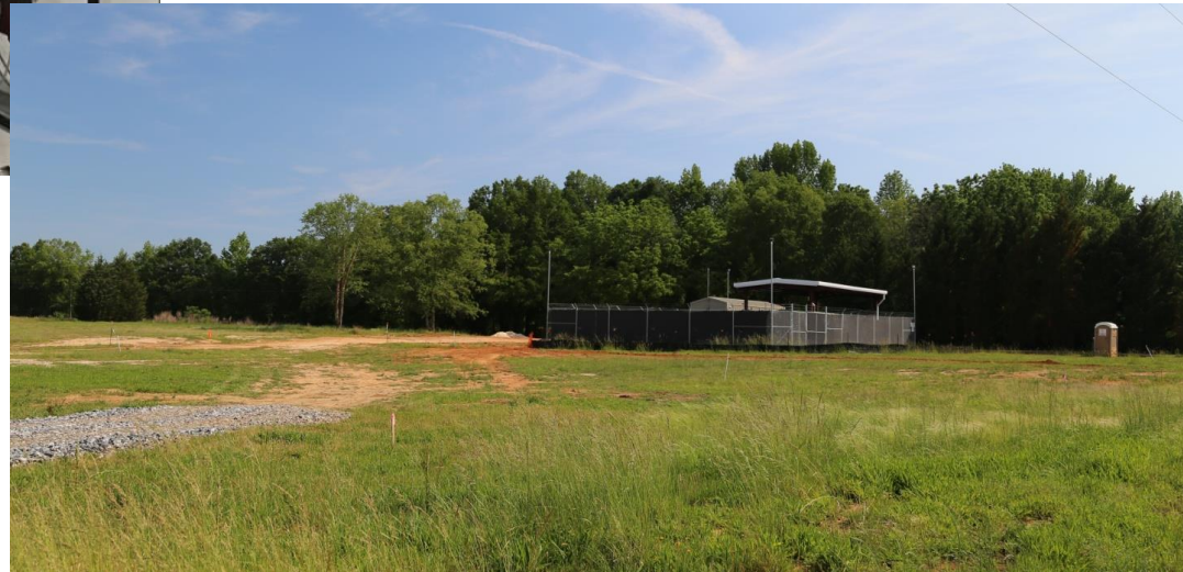
Biosparge Control Building- Street View
